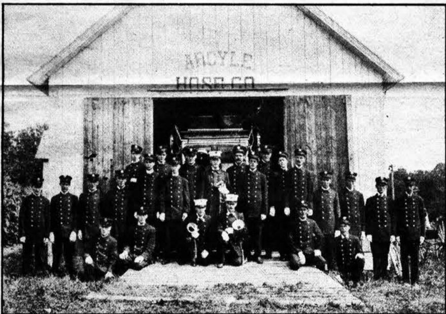
Argyle Hose Co. building, on Little East Neck Road, is still used.
