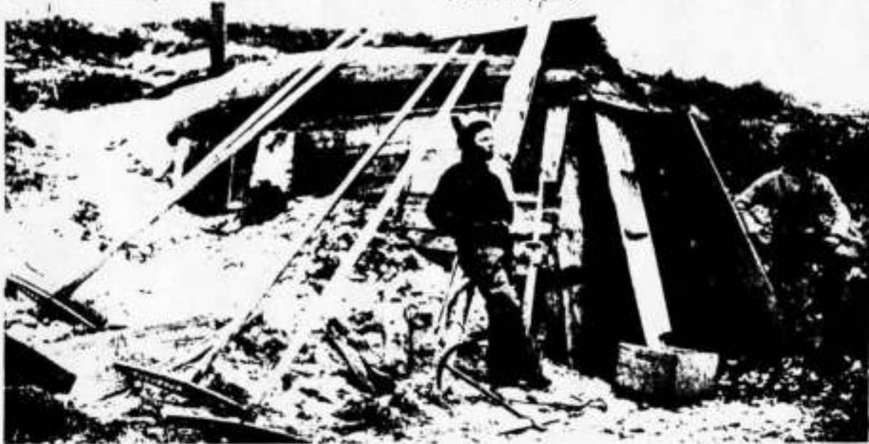
FIRE ISLAND "SQUATTER" SHACK, JULY 27, 1966
