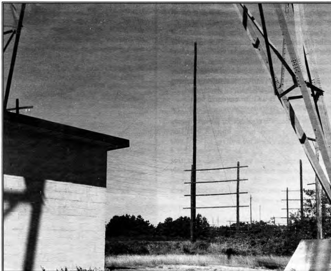
Base pedestal and one leg of the last remaining 410' tower at RCA Radio Central in Rocky Point. This 150 ton tower came down on Dec. 13, 1977. (photo and text courtesy of Robert Lundquist)
