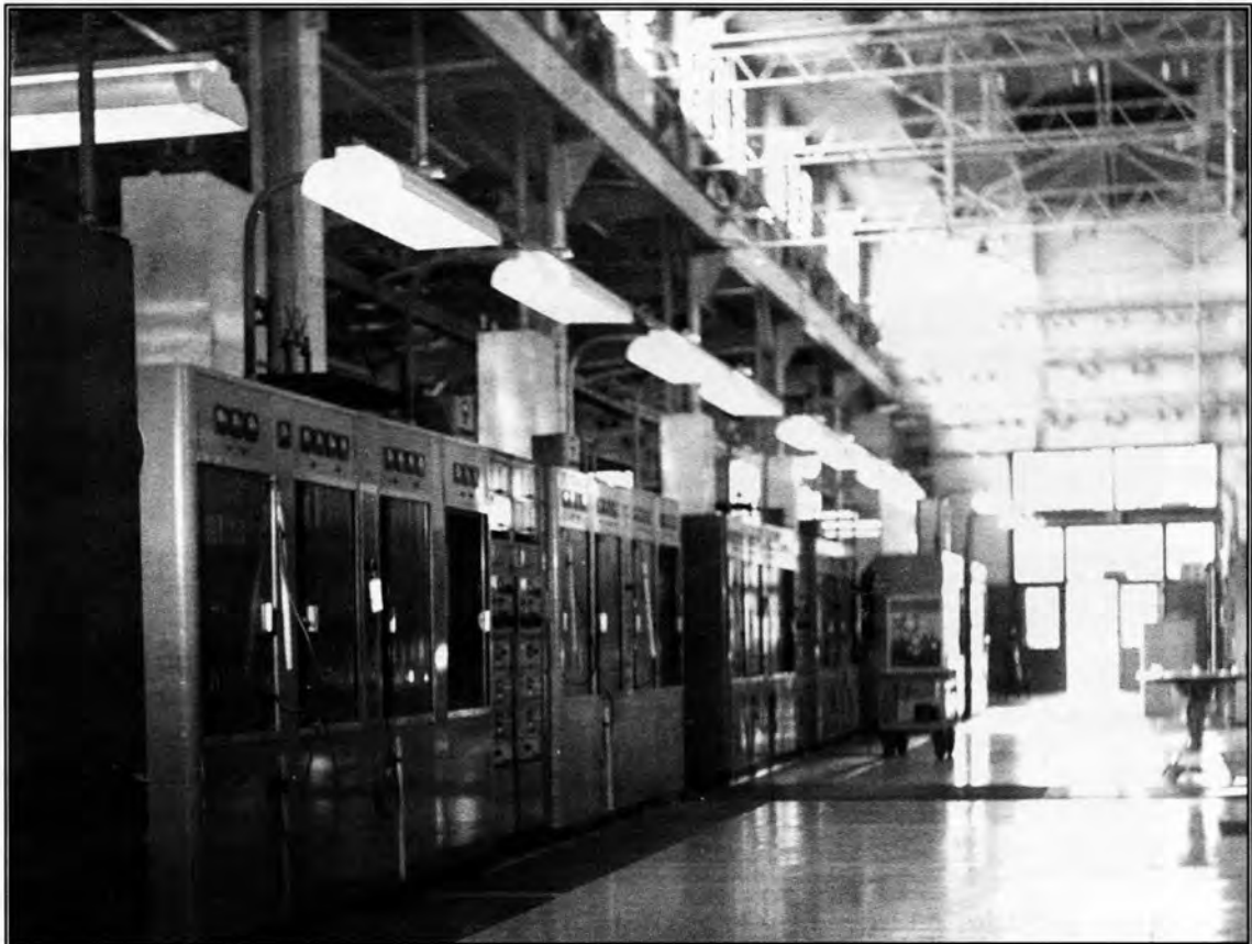
Interior view of Bldg. #1 looking southwest
