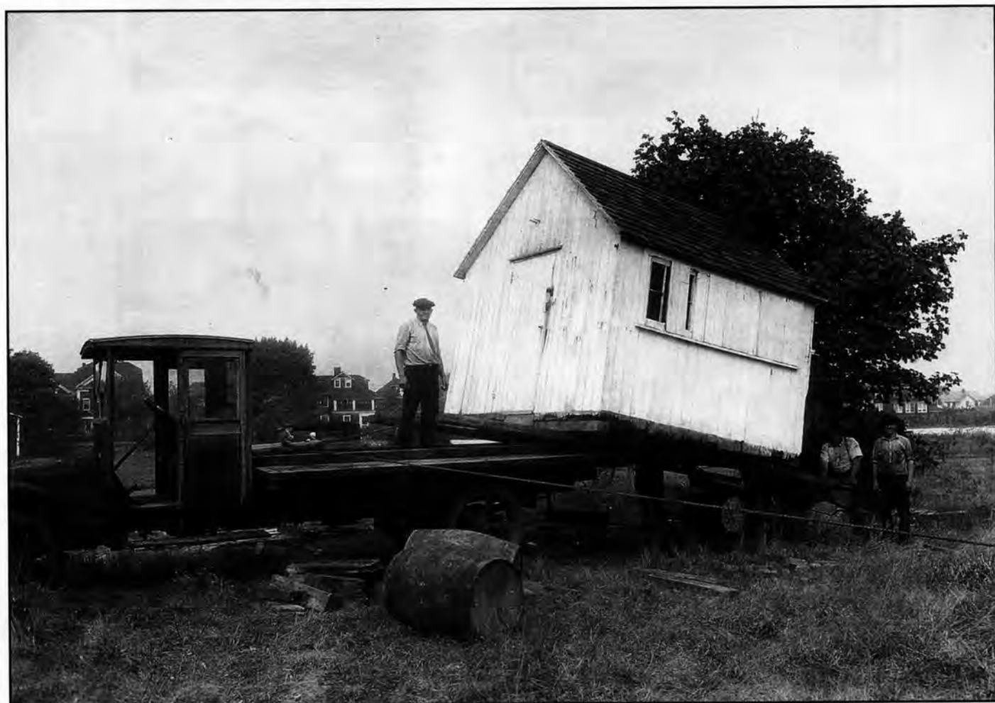
1930 - Loading the Marconi wireless station building to transport it from Babylon to the RCA Radio Central facilities in Rocky Point Photo by Thomas Coke Knight for Radio Corporation of America Courtesy David Sarnoff Library
