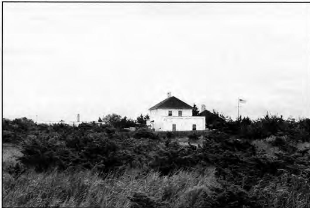
Above photo shows the rectangle original Telefunken Compass Building in foreground, and Barracks Building in background, now known as "Checkpoint" at Fire Island
