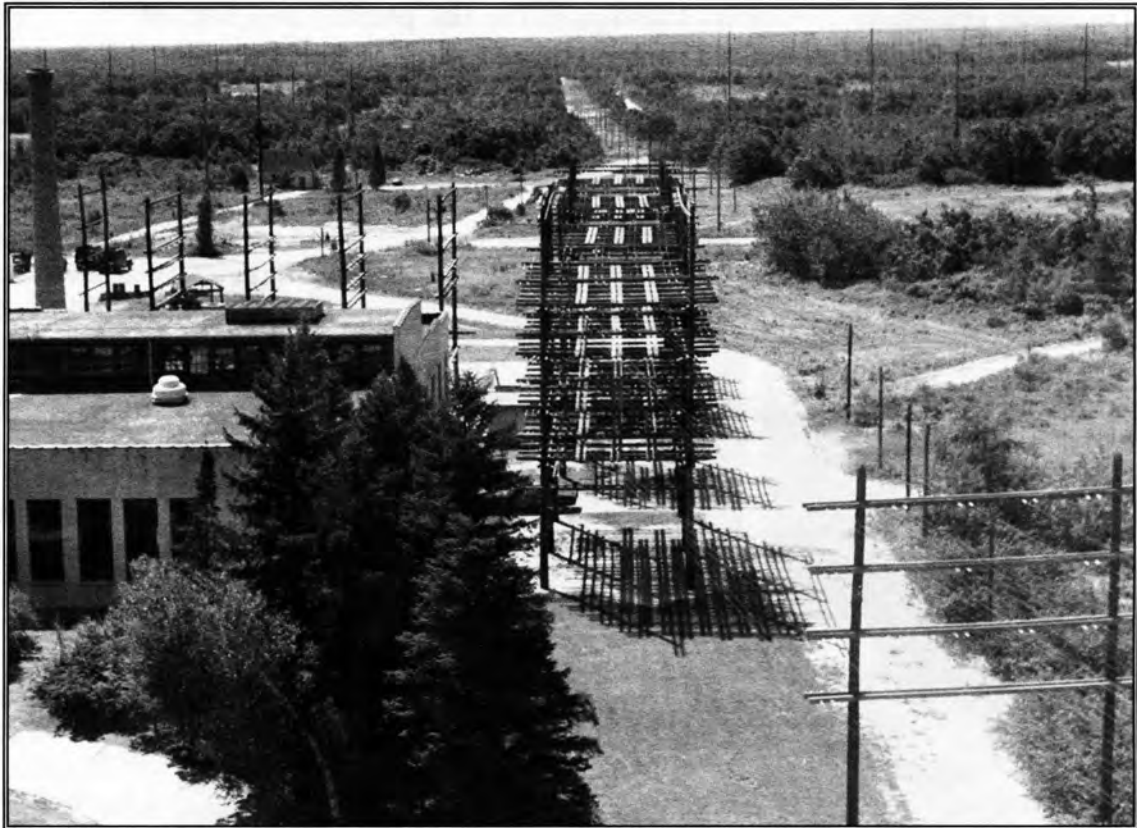
View of Bldg. #1 showing transmission trunk lines and southeastern section of antenna farm
